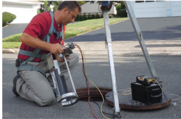
Figure 5: NIST traceable Billing Meter monitors flow from neighboring communities
