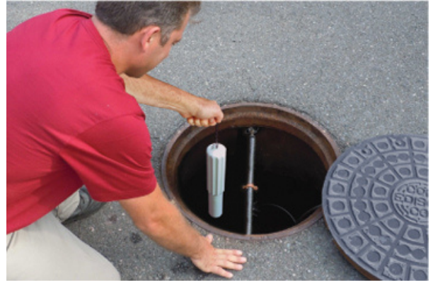
Figure 4: iTrackers become fully operational in 15 minutes without confined-space entry
